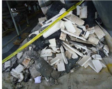
After insulation was removed the manifold is being high pressure water washed and also containing the area with monarflex.
