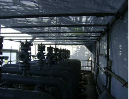
Picture shows where all items are wrapped and protected before the blasting commences to prevent equipment damages.
