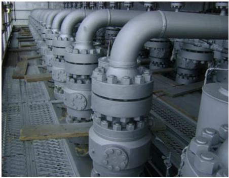
Fresh water washing the manifold after the primer coat application of Interplus 256 to remove any contaminants.
