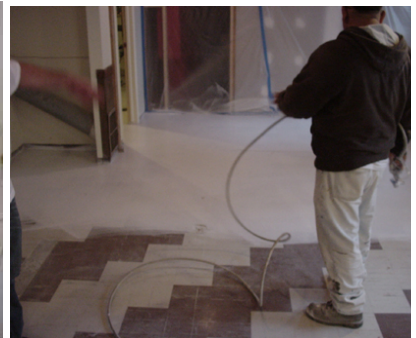
Painting floor thermal over cement
