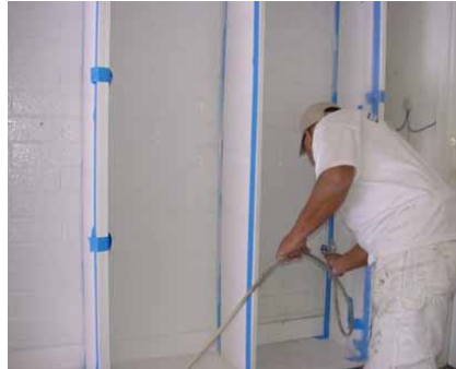
Painting un-insulated walls
